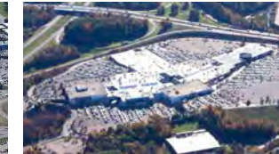
Galleria at Crystal Run Middletown, NY – 1,200,000 sf
